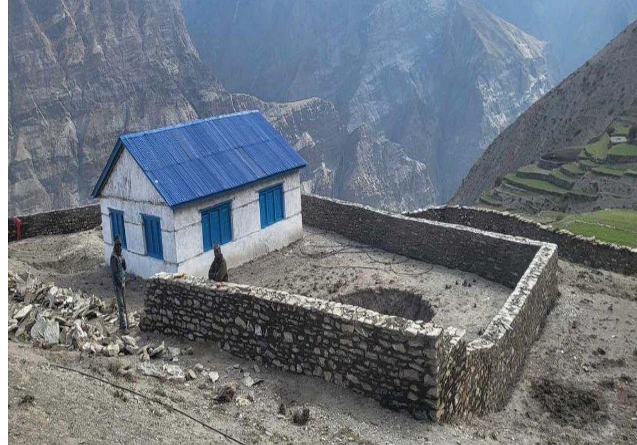
During septic tank and boundary wall construction
