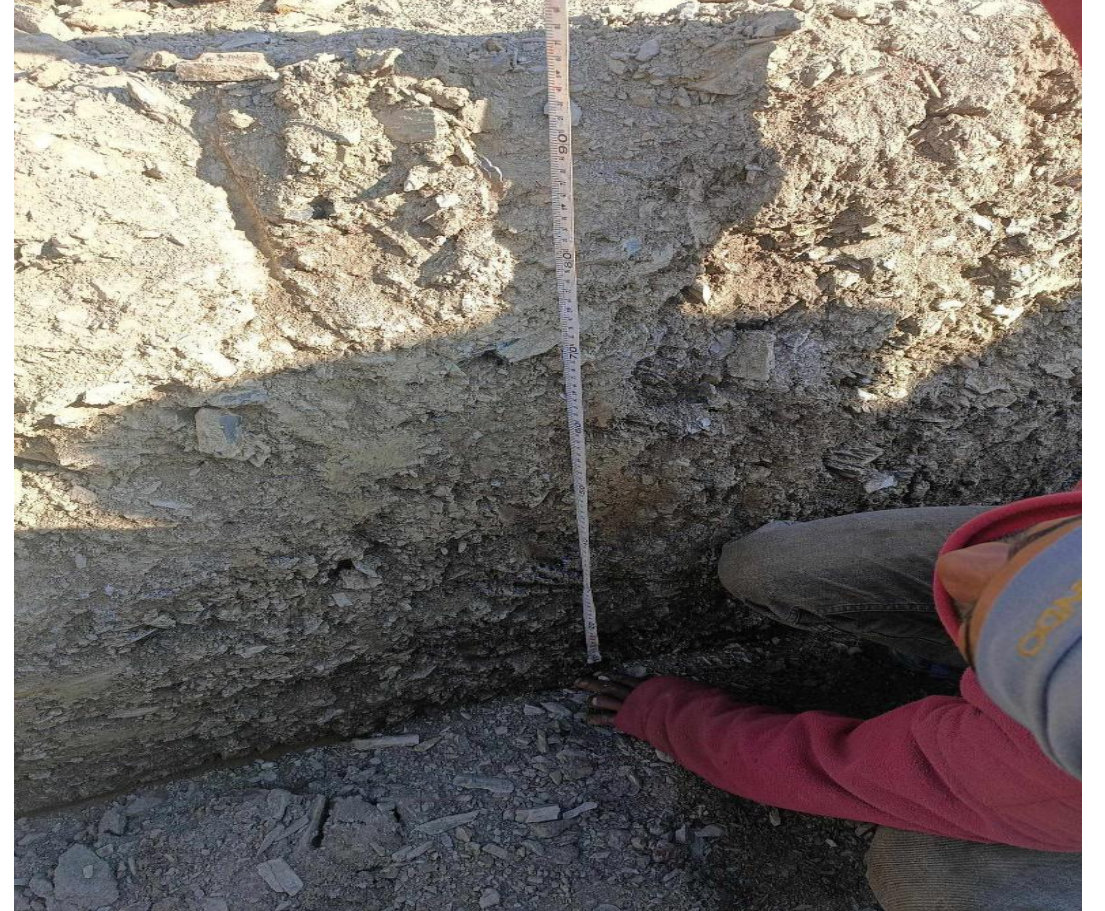
During foundation construction
