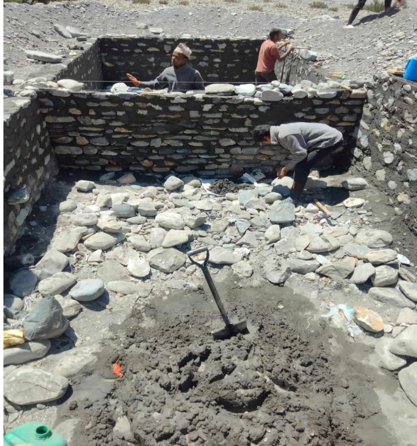
During dumping site and sewage chamber construction
